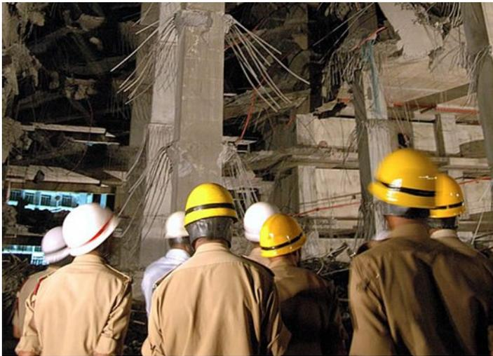
Fig 10: Flat Slab Bangalore Building Progressive Collapse—2008
