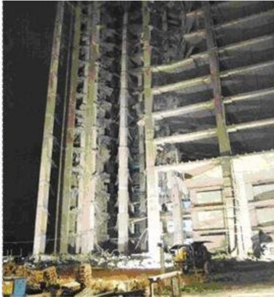
Fig 9: Flat slab Bangalore building progressive collapse-2008
