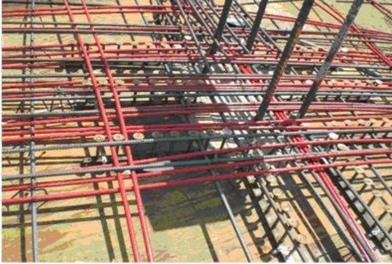
Fig 4. Typical Column-Slab Joint—USA East Coast Construction
