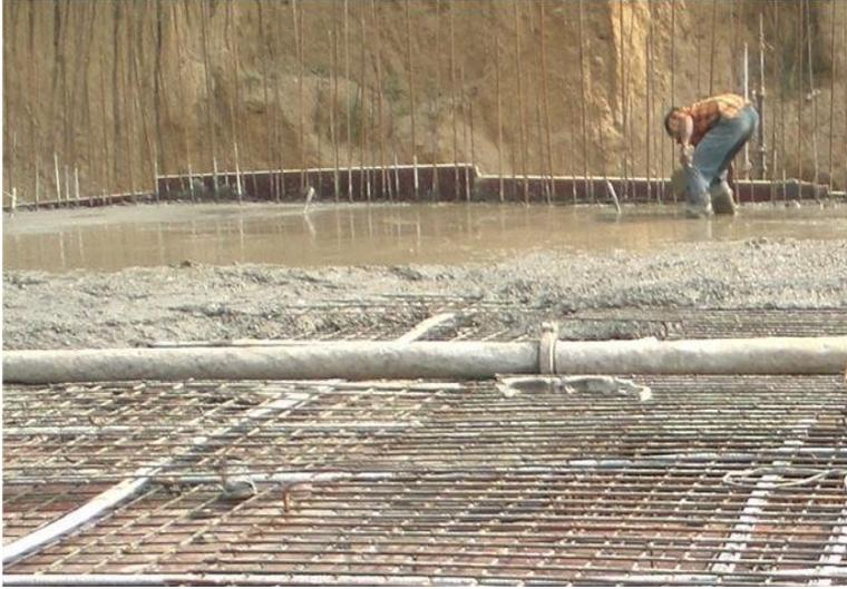
Fig 11: Shear Walls Being Cast Monolithically with PT Slabs!!!
