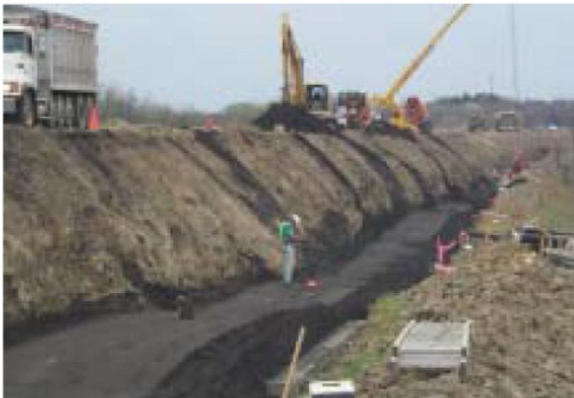
*Embankment with foundry sand subbase (Ohio Turnpike, sand from Ford Motor Company)*
