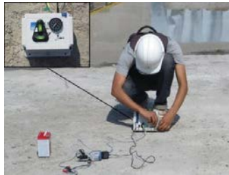
Fig.4–Leveling and Aligning of sensor on roof top
