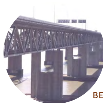
This bridge in California is near two active seismic faults, designed for 1.2 m of displacement and remain operational after a major earthquake
