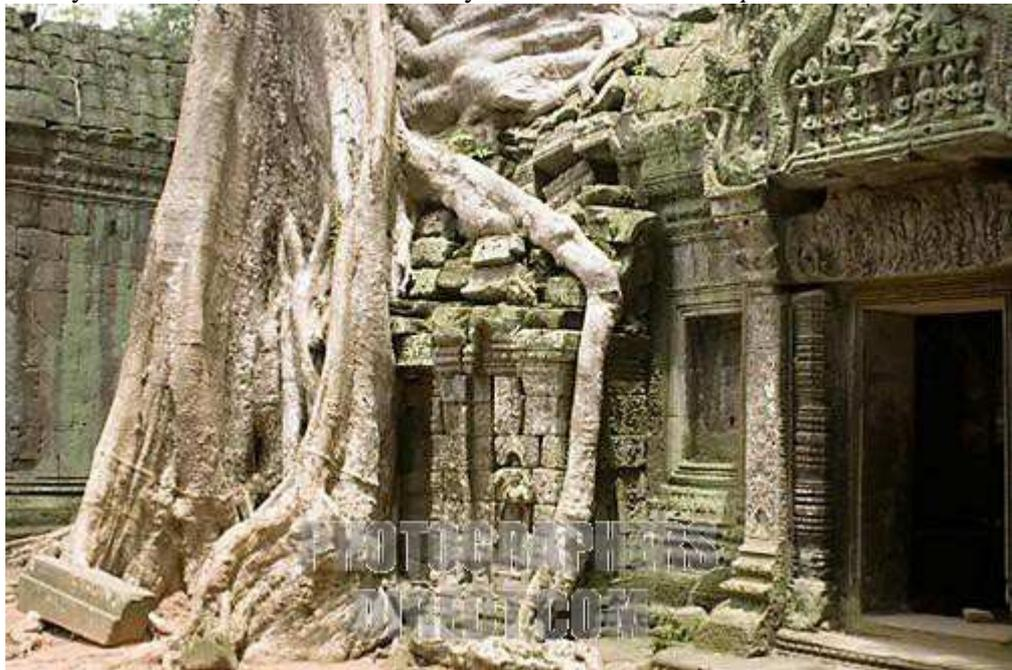
Fig. 23 – Large size tree trunk, barchnes, which have damaged the structure of the temple
