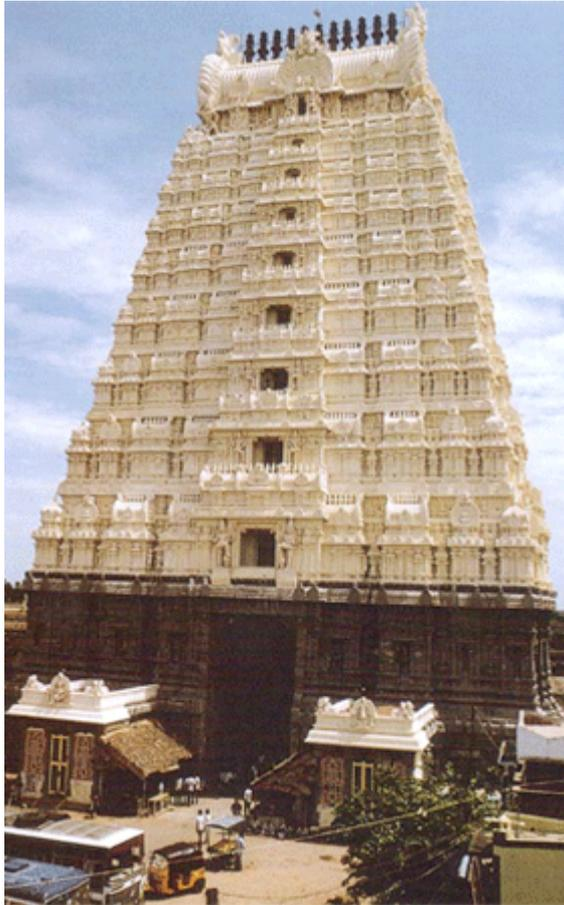
*Fig.1 – Typical ‘Shikhar’ of a South Indian Temple showing lowering of Centre of gravity, for better seismic response.*
