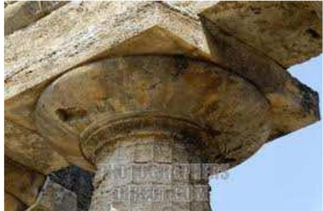
Fig. 14 – Column with circular corbel (something like what is done in a flat slab roof)
