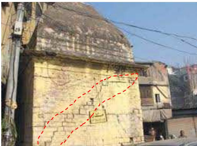
Fig.25 – Diagonal cracking in the Masonry wall of an Olden Temple
